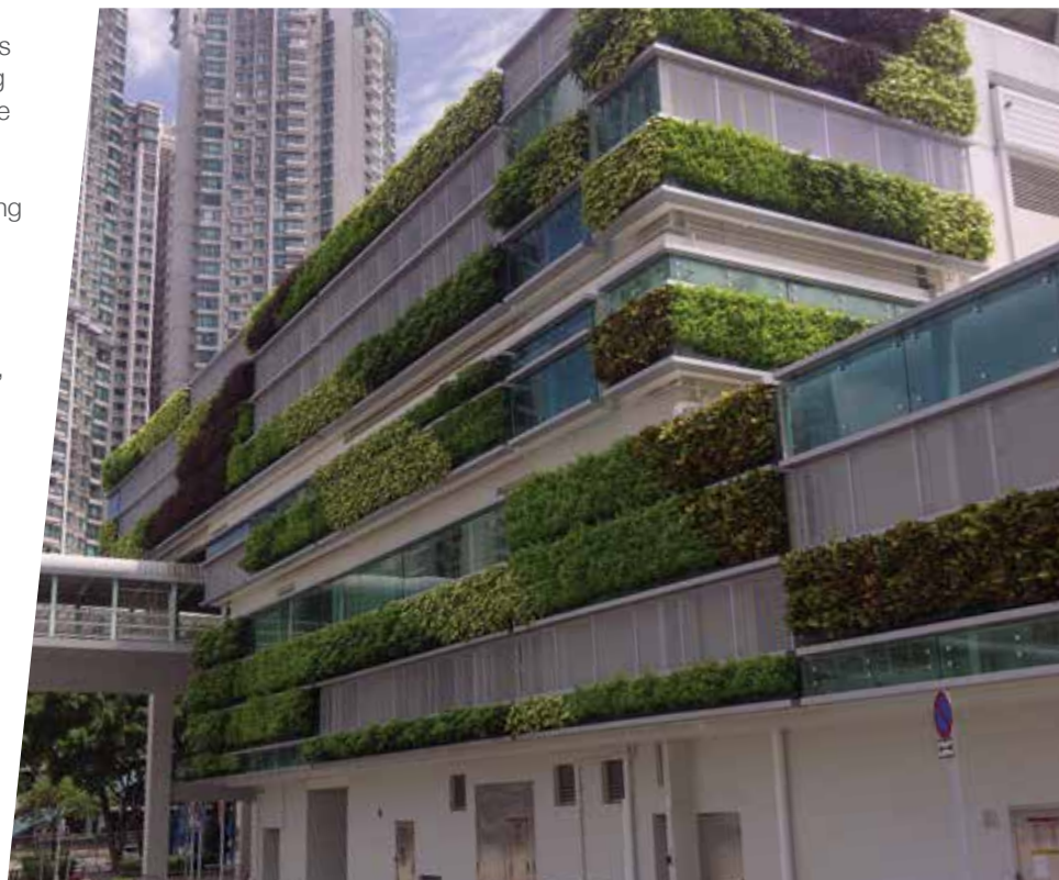
The New Energy Centre at Sha Tin Racecourse houses energy-efficient water-cooled air-conditioning systems.
